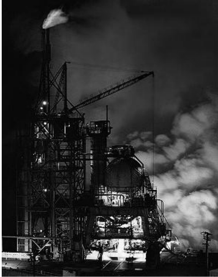
Figure C-3. Testing of SSME Solid Wall Hot Gas Manifold installed in Coca I Test Stand, SSFL, direction and date unknown.
